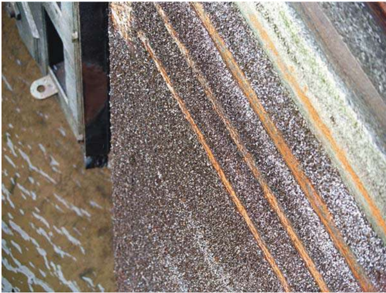
Figure 10: These zebra mussels, an introduced species, colonize most manmade and natural surfaces, including native mussels. Here they have infested the walls of the Arthur V. Ormond Lock, on the Arkansas River. They have caused significant damage to American waterways, locks, and power plants.
